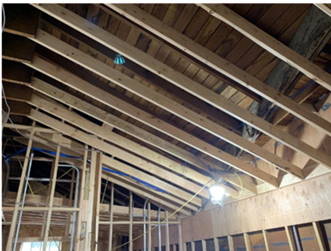
Level 2 Framing for Roof Insulation
