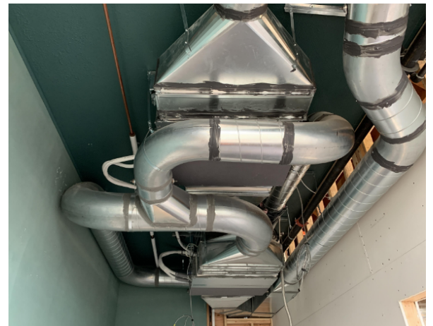
Level 1 HVAC Rought In and Drywall
