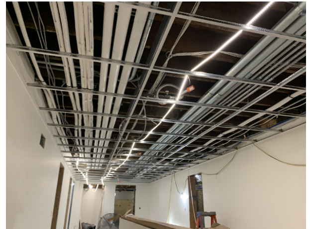
Installation of Ceiling Grid in Basement
